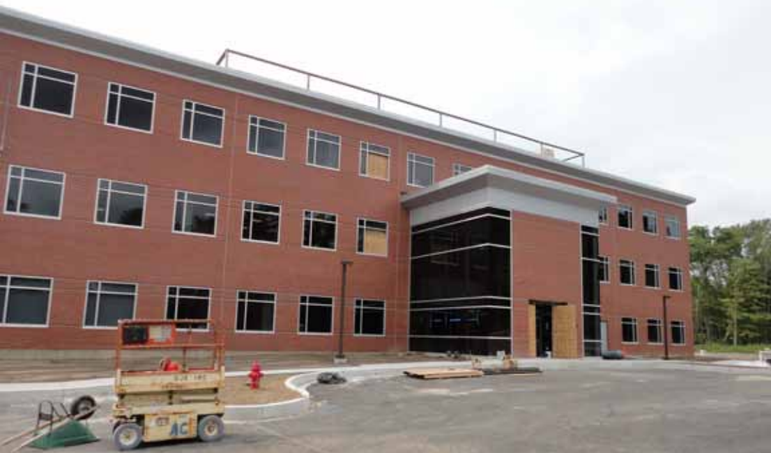
OUTER CONSTRUCTION, COMPASS MEDICAL MIDDLEBOROUGH, AUGUST 2011
