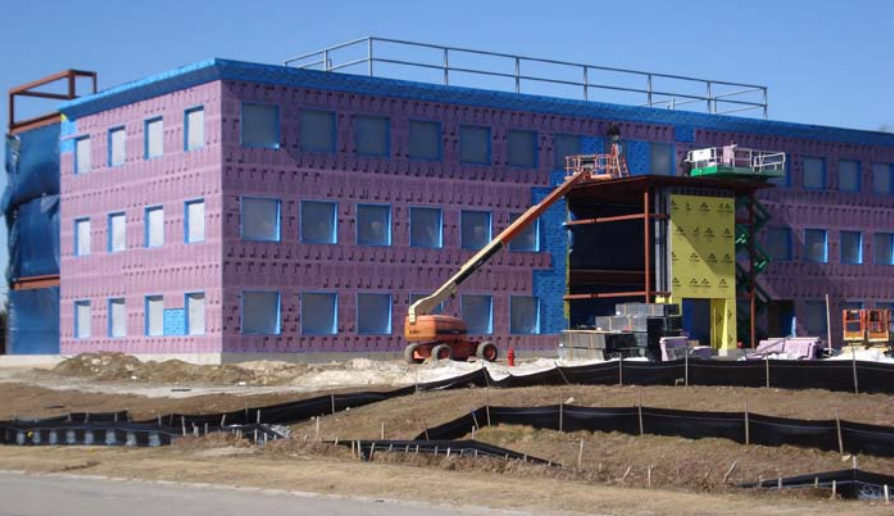
OUTER CONSTRUCTION, COMPASS MEDICAL MIDDLEBOROUGH, MARCH 2011
