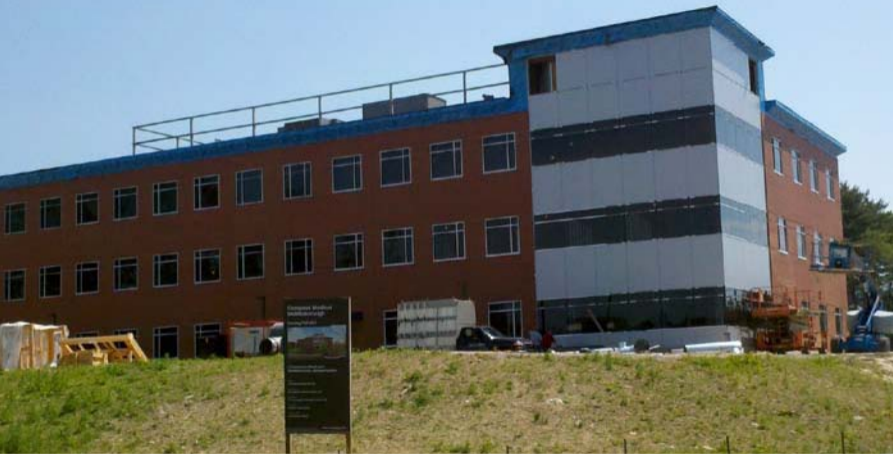
OUTER CONSTRUCTION, COMPASS MEDICAL MIDDLEBOROUGH, JUNE 2011
