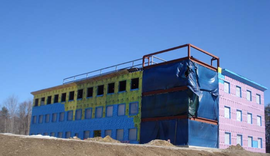
OUTER CONSTRUCTION, COMPASS MEDICAL MIDDLEBOROUGH, MARCH 2011
