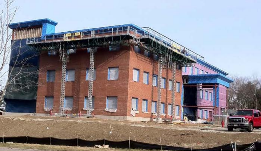
OUTER CONSTRUCTION, COMPASS MEDICAL MIDDLEBOROUGH, APRIL 2011
